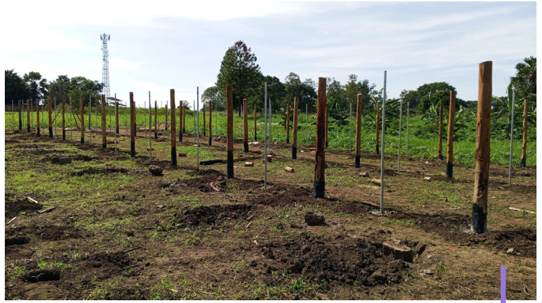
Photos from left to right: After the wind: the fallen greenhouse; rebuilding the first bay of the shade greenhouse
