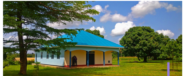
The new library is complete.
