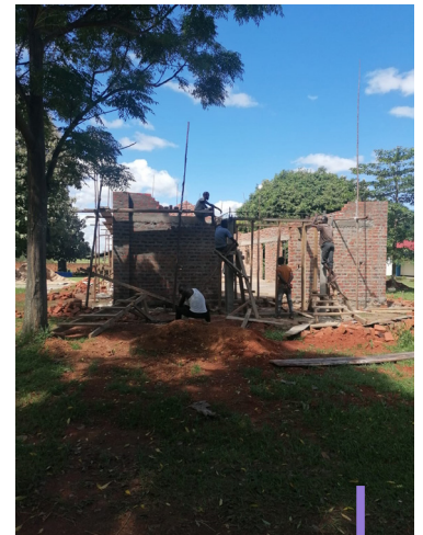
Photos from top to bottom: Breaking ground for the chapel with Pastor Kim (the donor), Barnabas (the works supervisor), Bishop Godfrey Loum (Bishop of the Diocese of Northern Uganda), Canon Willi Akena, two lay reader students and CT Wilson, the caretaker; the piggery almost ready for occupancy; the chapel in progress 15.11.23
